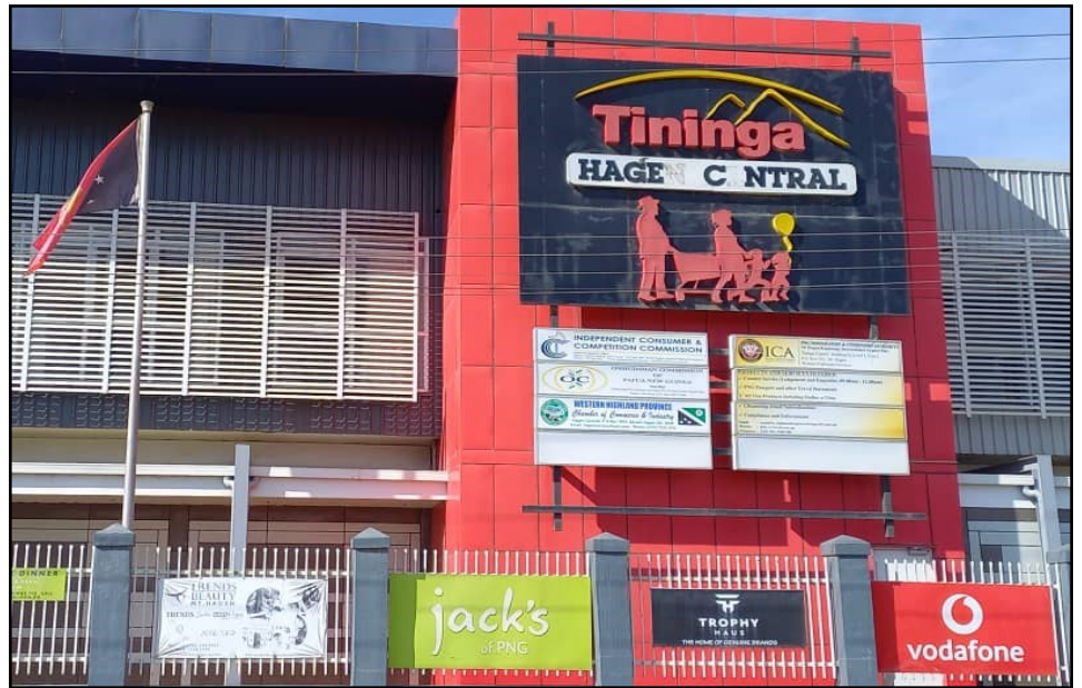
ICCC's Highlands Regional Office situated at the Tininga Central Building in Western Highlands Province.
